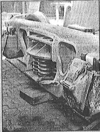
Second Generation Solid Bearing Truck
